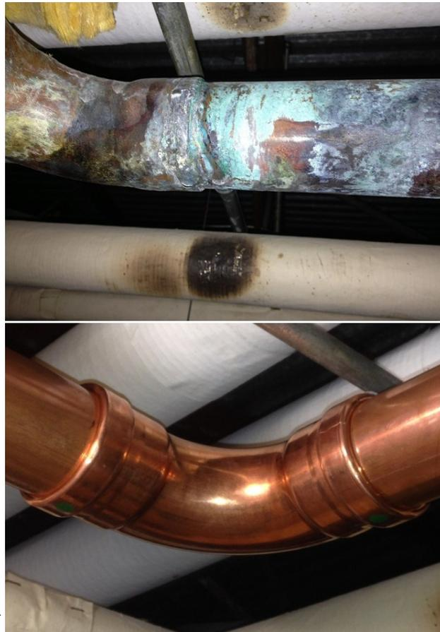
*Image 1—Before and after corrosion of main water pipe in East Tennessee Regional Health, Knoxville*
